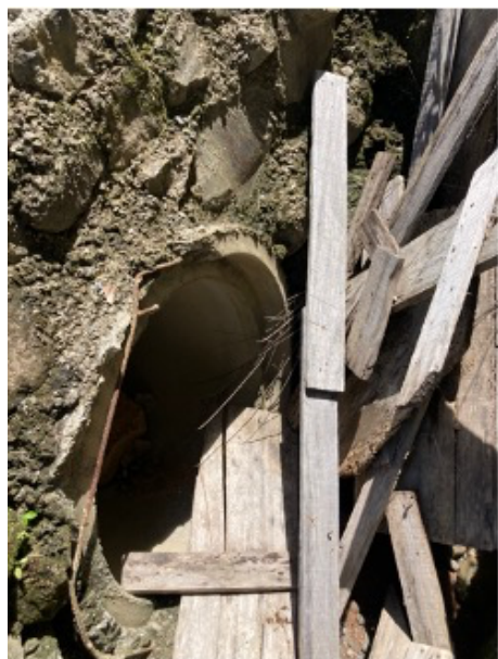
Appendix 7: Entrance of culvert 1. Wooden debris from cliff ladder shown.
