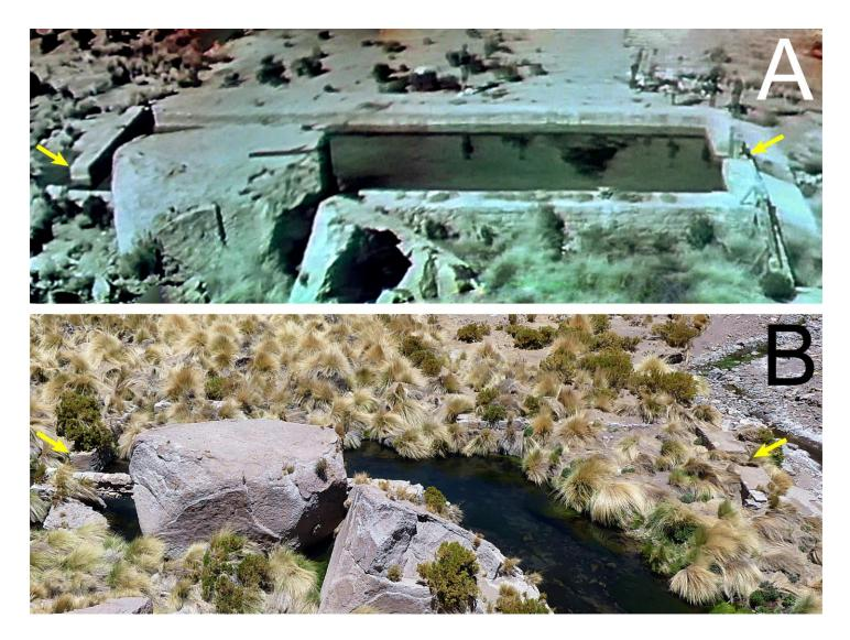
**Figure 3.** Historic and current state of the concrete swimming pool in Miño. **A** Panorama extracted from video footage from the IHAEC, 1935. Yellow arrows indicate the upper and lower pool walls. **B** Same view in 2020.
